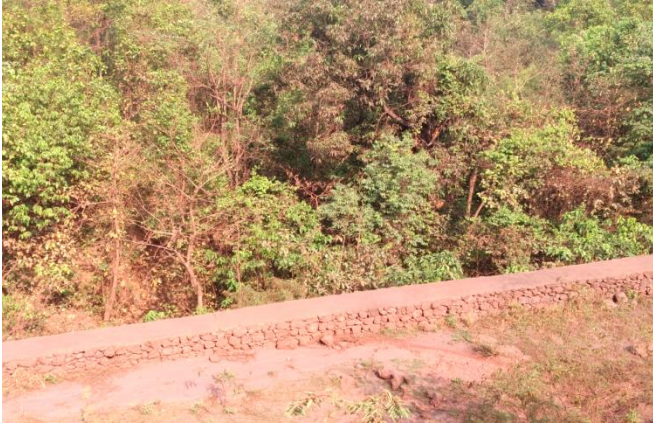
Photo-10: Check Weir
