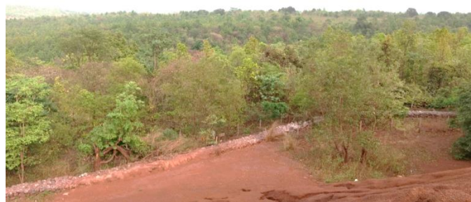
Photo-2 &3: Retaining wall along with Plantations at the toe of dump slopes
